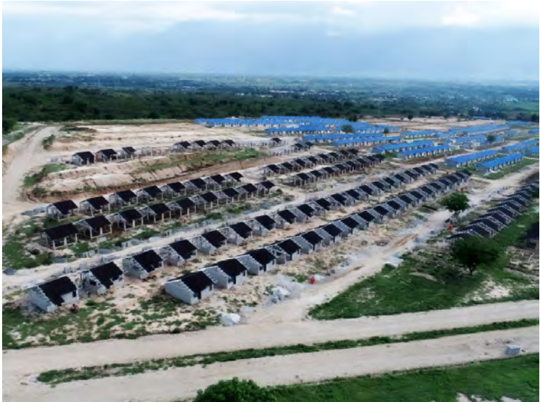
Huntap Pombewe while still under construction. The total number of huntaps in Pombewe is 1,117, of which 605 were built by the Ministry of PUPR. (Photo: Ministry of PUPR Documentation)
