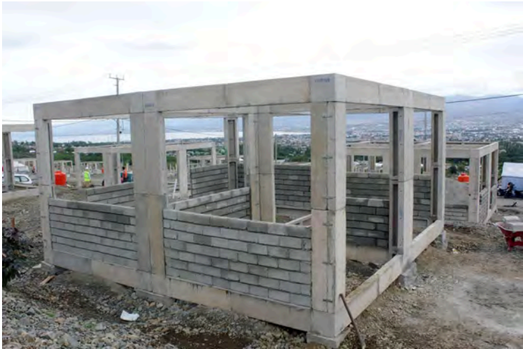
Model of RISHA's appearance at the Huntap Duyu site while still under construction. (Photo: The Ministry of PUPR)
