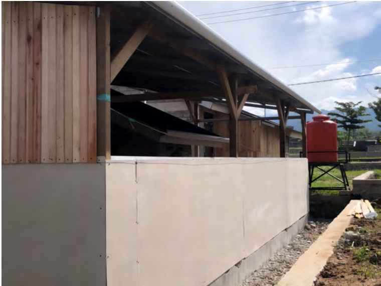
The construction of the kitchen in the Muli's huntap, a resident of Huntap Pombewe. Muli built his kitchen with semi-permanent materials to comply with the regulations. In the first year after the handover, residents were only allowed to develop their Huntap with semi-permanent materials. (Photo: Nur Rizky/The Ministry of PUPR)
