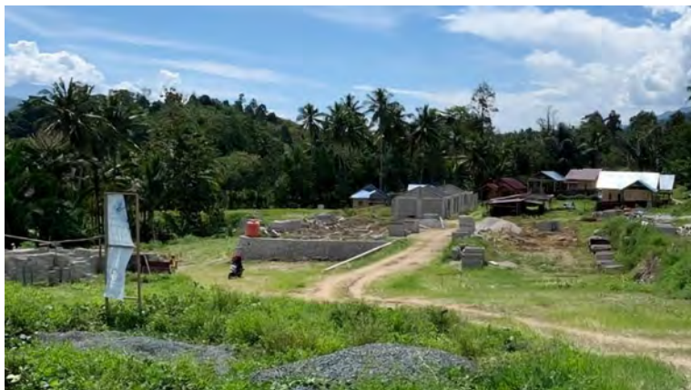
Huntap Salua while still under construction. The land that can be used in this site is only 14,463 m 2 for 63 units. With the availability of existing land, the plot per huntap unit in this site is only 8m x 12m, much smaller than it should be, which is 10m x 15m. (Photo: El/Special)
