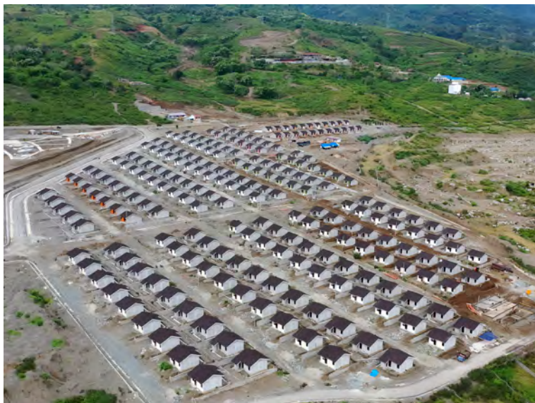
Huntap Duyu, Palu City, while still in the process of completion. Huntap Duyu occupies an area of 14.1 ha., built as many as 230 units, and is intended for the DAPs from 11 sub-districts in Palu City. (Photo: The Ministry of PUPR)
