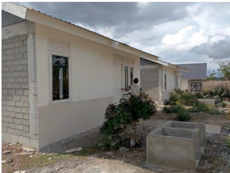
After going through a fairly long process to resolve land legality issues, these three huntap units were finally built and completed in early 2022. (Photo: Hadija/The Ministry of PUPR)
