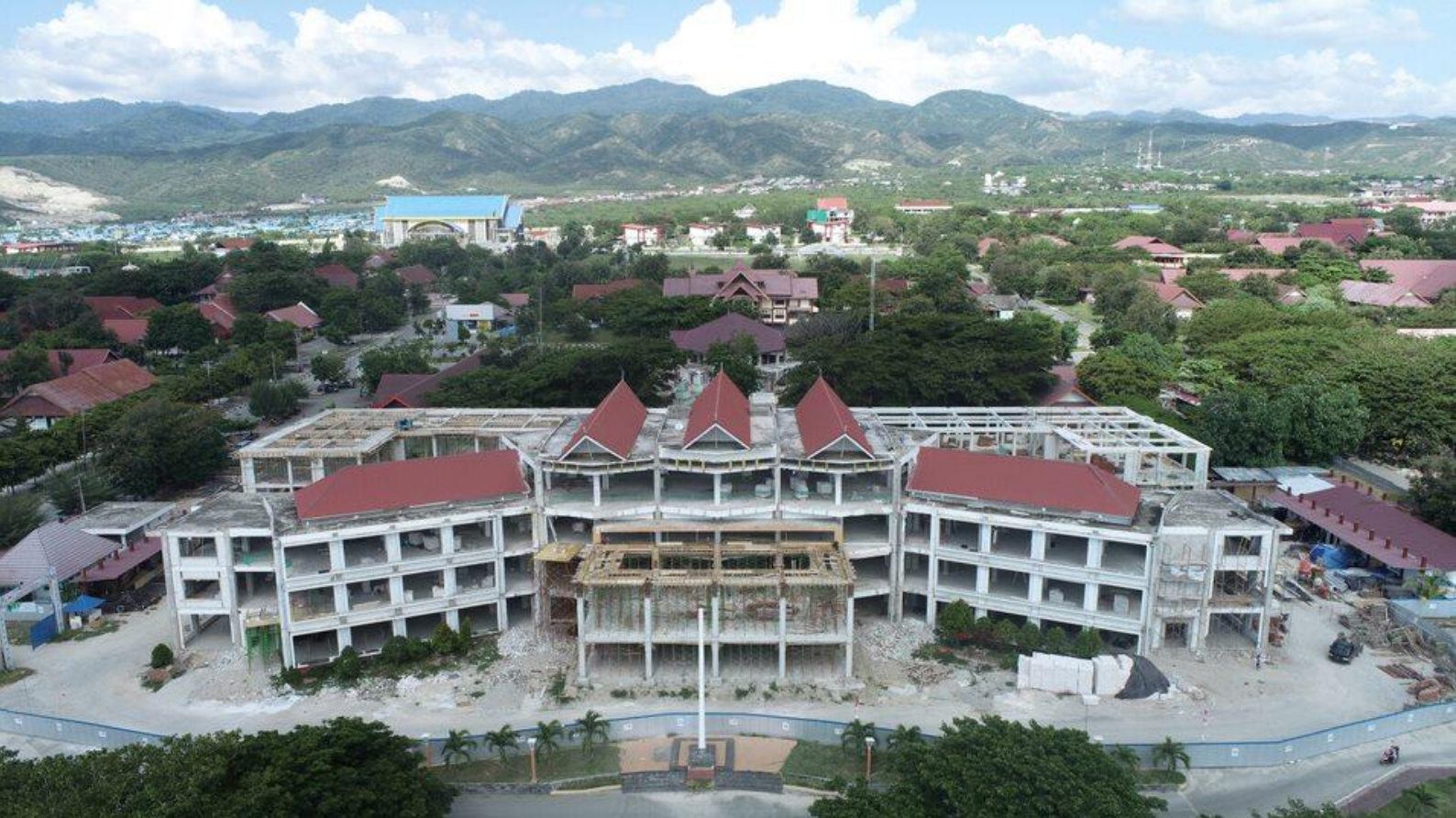
Tadulako University's rectorate building is being constructed in Palu, Central Sulawesi, on April 2023 (PMC/Aji Wahyu)
