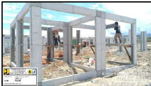
Pek. Penginstalan Panel Risha
