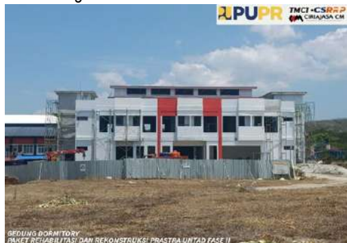
Progres Gd. Dormitory
