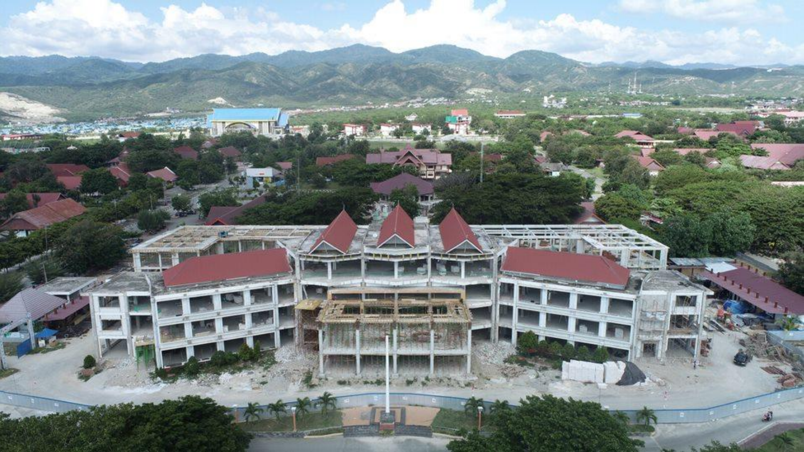
Tadulako University's rectorate building is being constructed in Palu, Central Sulawesi, on April 2023 (PMC/Aji Wahyu)
