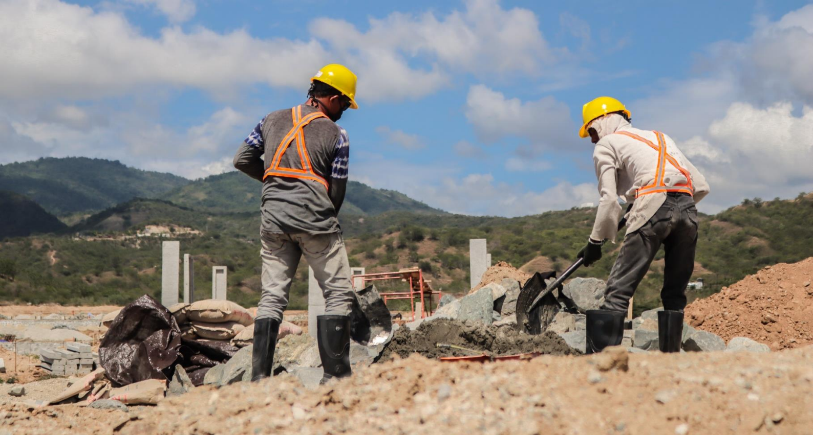
Two workers are picking up materials in Huntap Tondo 2 area (PMC/Haerul Fikri)
